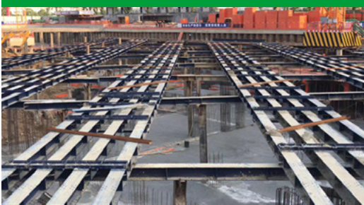
Steel Support System for Foundation Pit 基坑钢支撑体系
