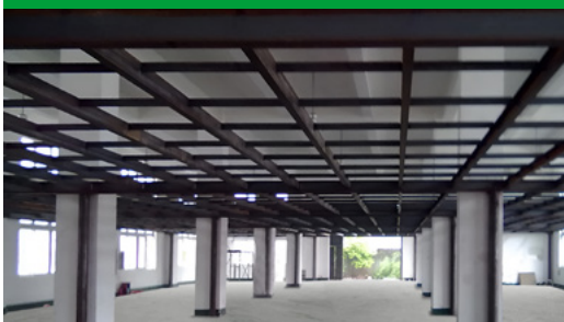
Steel Structure Mezzanine 钢结构夹层
