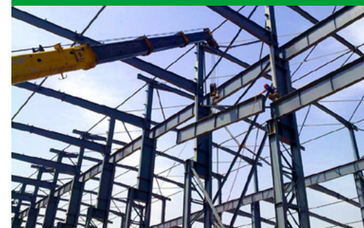
Light Steel Factory Building 轻钢厂房
